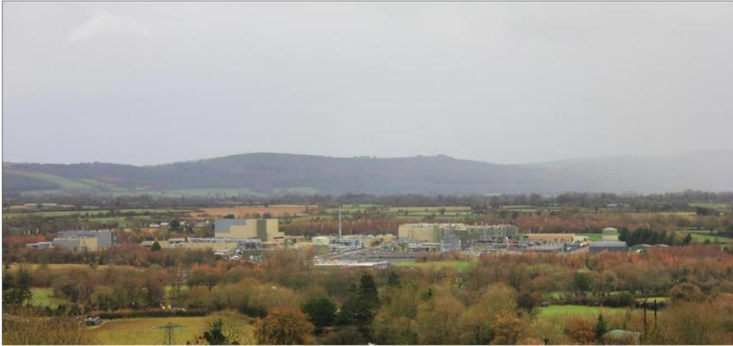
MSD Pharmaceutical Facility, Clonmel
