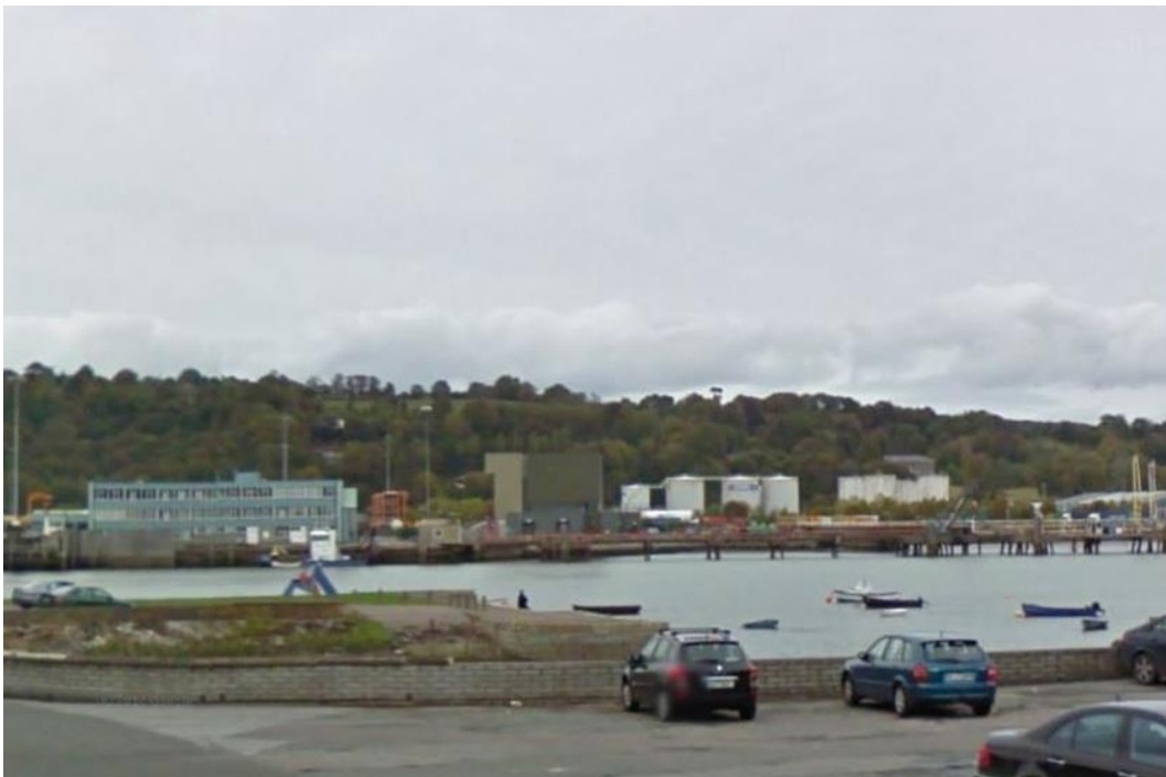
Port of Cork, Crane Maintenance building.
